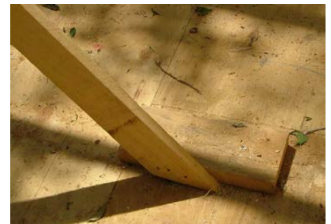
Figure 2. Nail your bracing to a block that is nailed to a joist.
