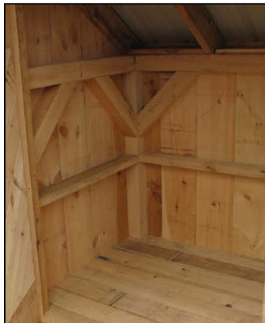
Figure 7 4x4 Corner bracing
