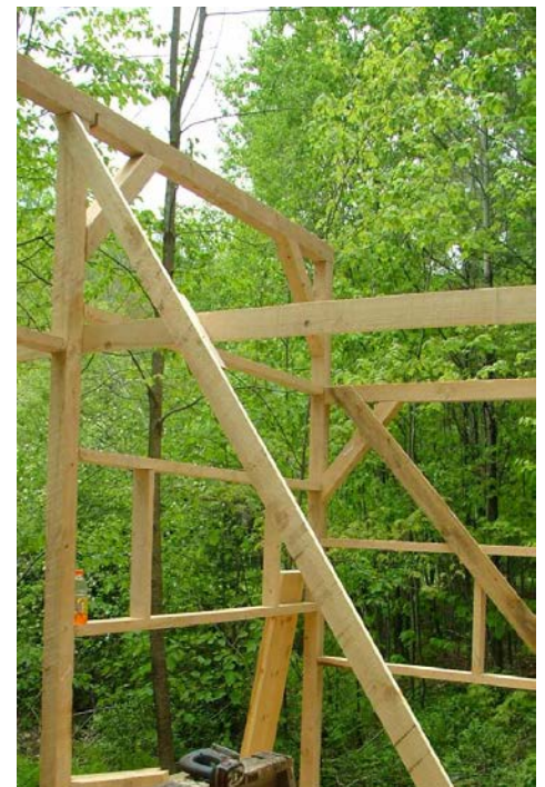
Figure 2. Nail your bracing to a block that is nailed to a joist.
