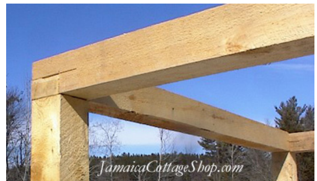
1/2 lap 4x4 top plate corner attachment
